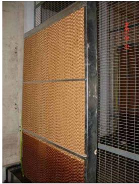
Cellulose pads of fan-pad cooling system for poultry
